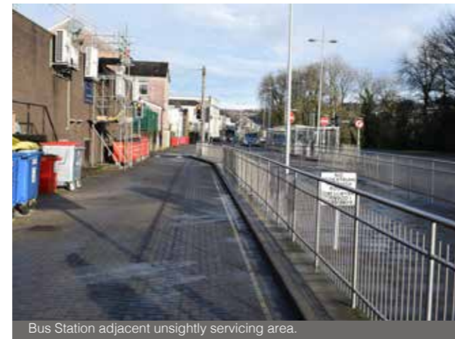
Bus Station adjacent unsightly servicing area.
