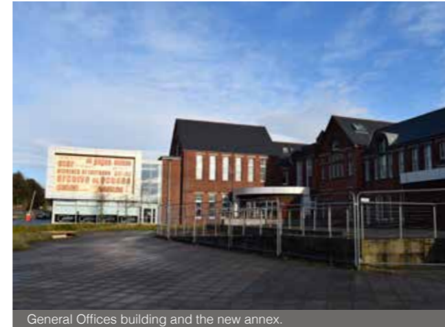
General Offices building and the new annex.
